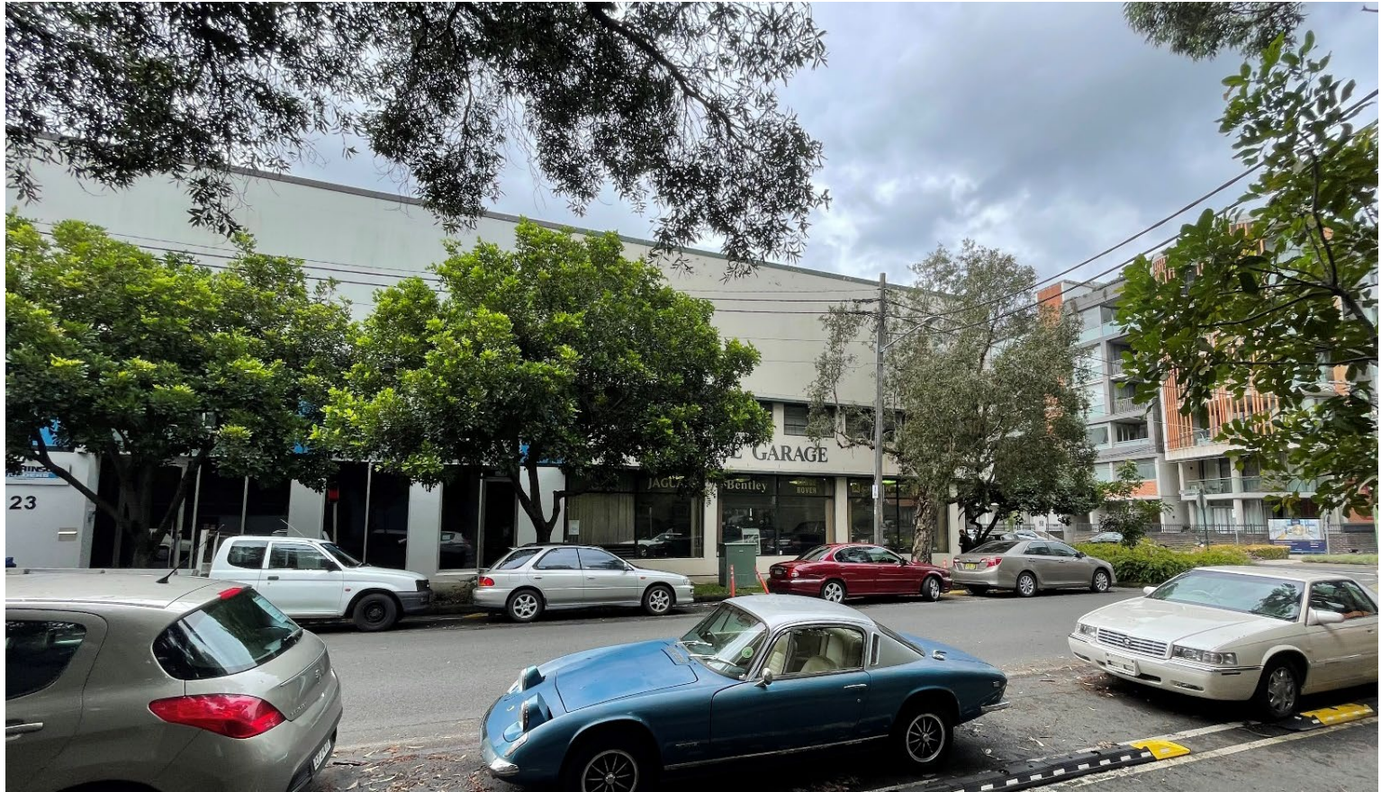
Dunning Avenue frontage
